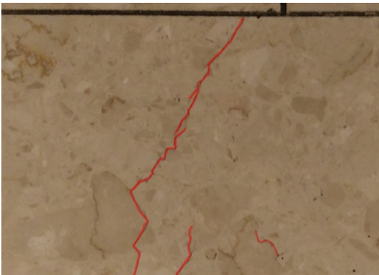
An example of tile cracks marked with high precision.
